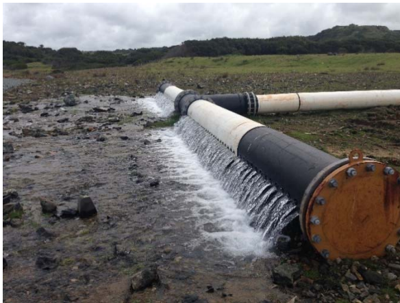
Water discharge during dewatering
