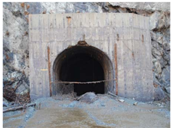
Underground portal when mine ceased production
